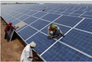
Installation of solar panels in a solar park in Charanka, India.
